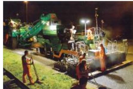
The temperature profiling has enabled the contractor to measure the extent of variability in surface temperature and hence draw a number of conclusions about temperature homogeneity. The monitoring of equipment movements using GPS systems has highlighted a number of operational issues. A number of benefits are apparent. The consequences of on-site operational behaviour and discontinuities are made explicit. The temperature profiling highlights the resultant variability in temperature
