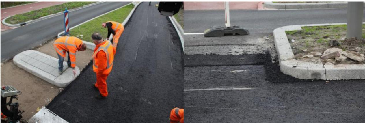
**Figure 1 and 2:** Manual asphalt spreading is needed at a refuge.
