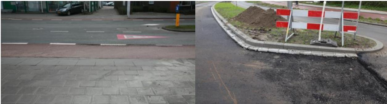
**Figure 3 and 4:** Longitudinal joints between different colored asphalt. First failure is visible (left). Segregation is clearly visible at a refuge (right).
