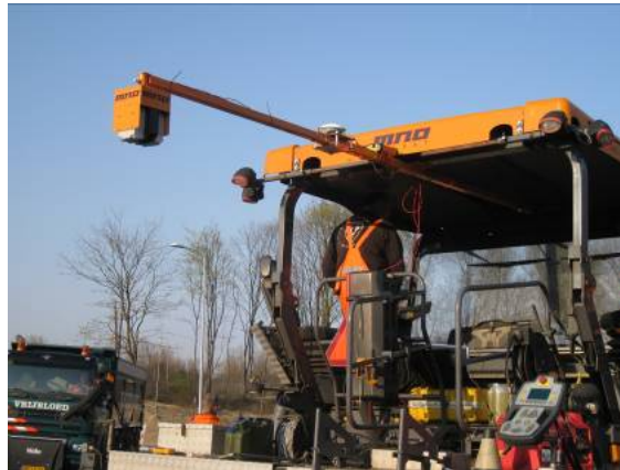
Figure 2: Linescanner mounted behind a paver
