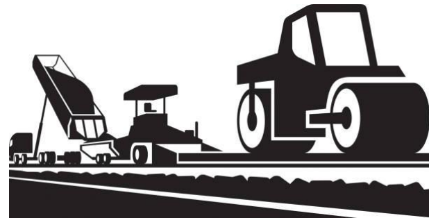
Asphalt placement and roller compaction
