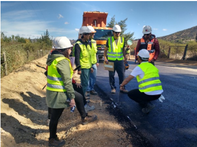
Project engineers on site
